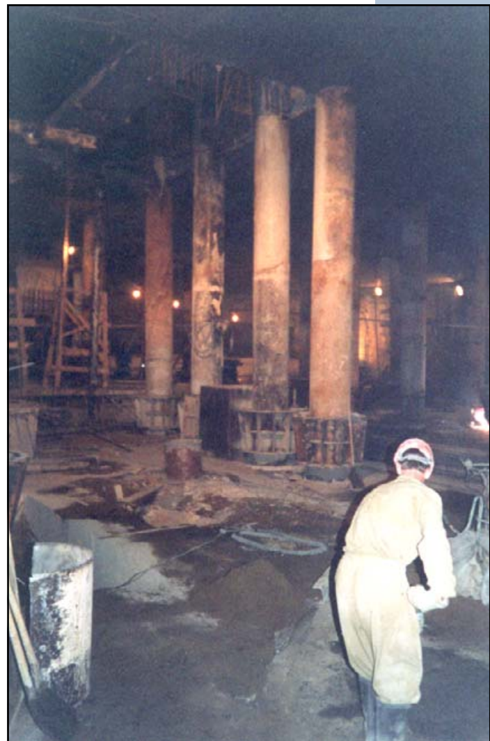
Fig. 2. Building 1. Construction of foundation slab in the zone of lift shafts.
