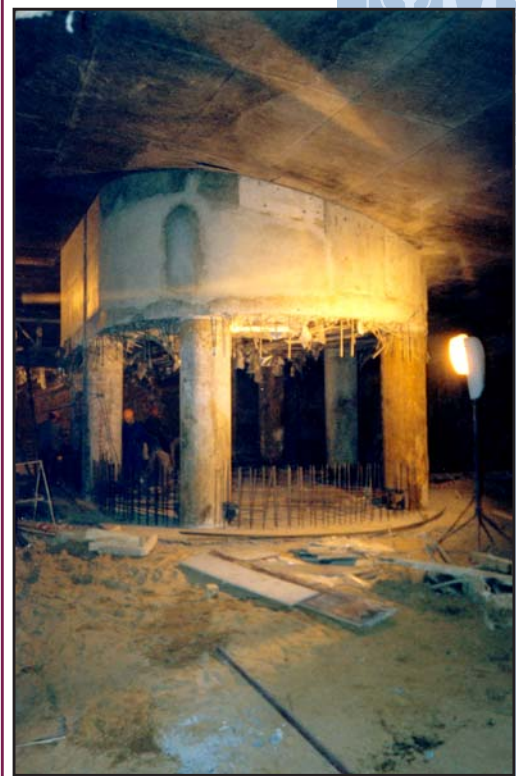
Fig. 9. «The Alfa-Arbat-Center» multifunctional complex in Moscow. View of the parking-garage western half -3 rd storey ramp central core structures «suspended» on bore columns before erecting the -4 th storey ramp.
