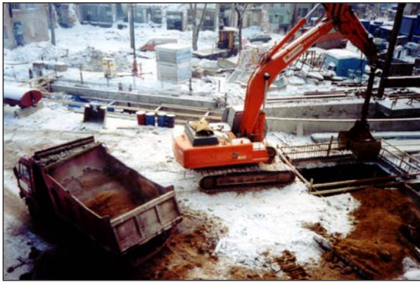
Fig. 11. «The Alfa-Arbat-Center» multifunctional complex in Moscow. Hitachi EX300-5 clamshell excavator working through temporary erection opening and bringing muck to the surface to be loaded into dump trucks while excavating 2 nd tier of the pit.
