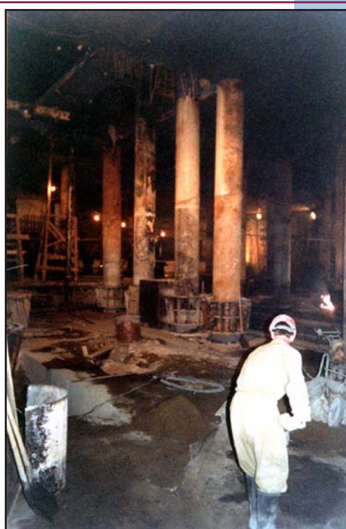
Fig. 2. «The Tsar's Garden» multifunctional complex in Moscow. «Suspended» on bored columns are lift and ventilation shafts of the Building 1 eight-storey aboveground part rigidity core.
