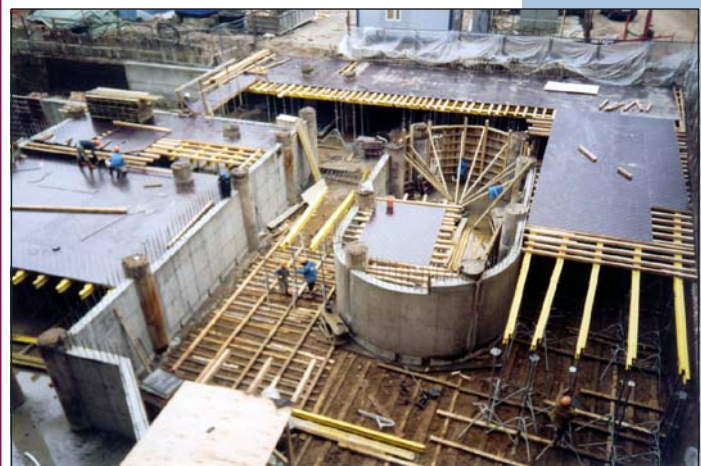
Fig. 8. «The Alfa-Arbat-Center» multifunctional complex in Moscow. View of the parking-garage western half -1 st storey ramp after erection of the central core walls and external ramp fire-fighting walls before laying the roof-slab.
