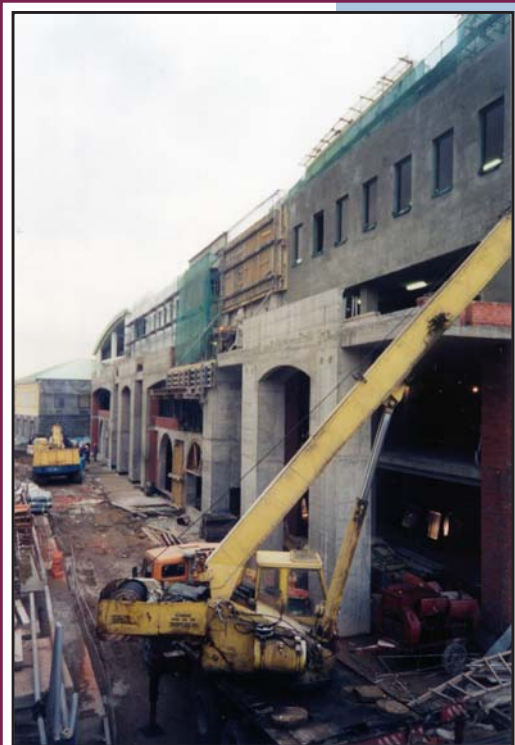
Fig. 4. «The Tsar's Garden» multifunctional complex in Moscow. Erecting Building 1 face walls.
