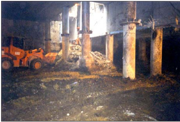
Fig. 15. «The Alfa-Arbat-Center» multifunctional complex in Moscow. Excavation in the 4 th tier of the pit in the parking-garage eastern half ramp area.
