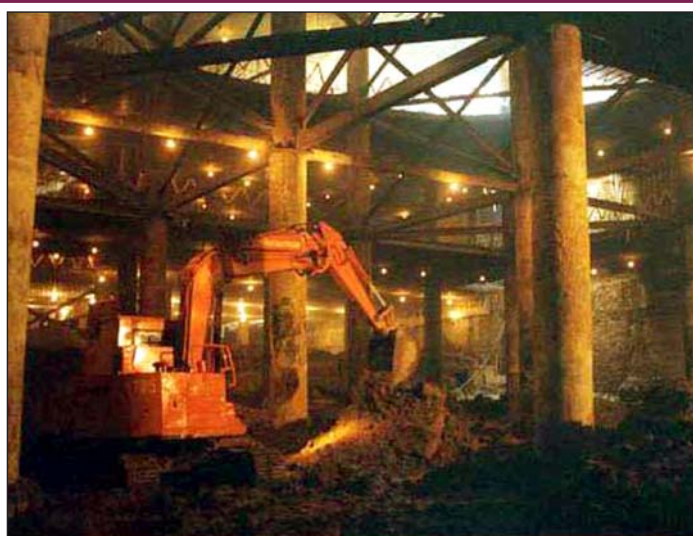
Fig. 3. «The Tsar's Garden» multifunctional complex in Moscow. Temporary steel support structure to fill openings in floor-slabs of the Building 1 underground part at the access ramp place.
