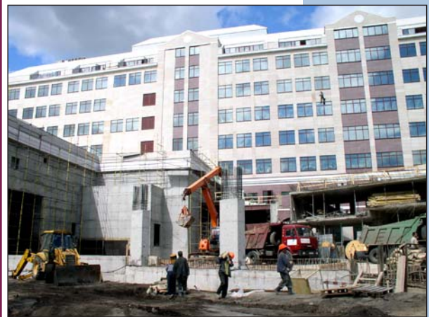
Fig. 18. «The Alfa-Arbat-Center» multifunctional complex in Moscow. Completing construction of the extension to the main building. Erecting structures of the third stage construction package over the underground parking-garage eastern half while excavating the 5 th tier of the pit.
