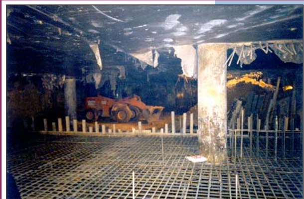
Fig. 19. «The Alfa-Arbat-Center» multifunctional complex in Moscow. Completing excavation of the 5 th tier of the pit near the erection opening.
