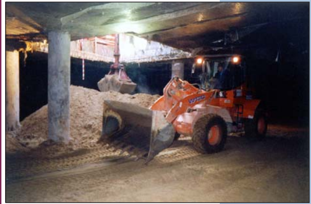
Fig. 12. «The Alfa-Arbat-Center» multifunctional complex in Moscow. Hitachi W130 motor loader transporting muck to temporary erection opening while excavating the 2 nd tier of the pit. Muck is brought to the surface using Hitachi EX300-5 clamshell excavator and loaded into dump trucks.
