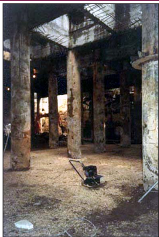
Fig. 5. «The Tsar's Garden» multifunctional complex in Moscow. «Suspended» on bore columns are lift and ventilation shafts of the Building 3 eight-storey aboveground part rigidity core.
