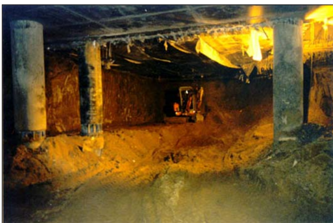
Fig. 13. «The Alfa-Arbat-Center» multifunctional complex in Moscow. Excavation in the 3 rd tier of the pit under the parking-garage western half -2 nd storey ramp.
