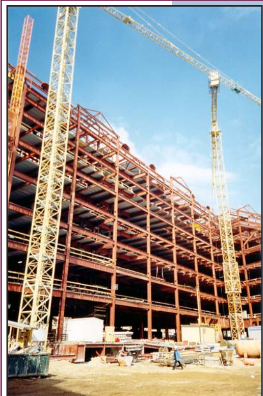
Fig. 6. «The Alfa-Arbat-Center» multifunctional complex in Moscow. Erecting main building steel bearing framework after completion of underground parking-garage diaphragm walls.
