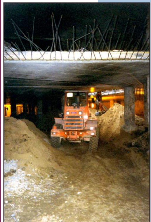
Fig. 14. «The Alfa-Arbat-Center» multifunctional complex in Moscow. Hitachi W130 motor loader transporting muck to temporary erection opening while excavating the 3 rd tier of the pit under the parking-garage western half -2 nd storey ramp.
