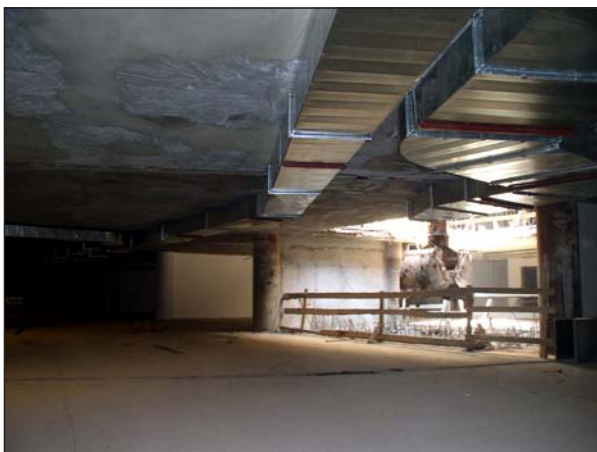
Fig. 17. «The Alfa-Arbat-Center» multifunctional complex in Moscow. Installing ventilation and fire-fighting permanent systems at the -2 nd storey while excavating the 5 th tier of the pit.
